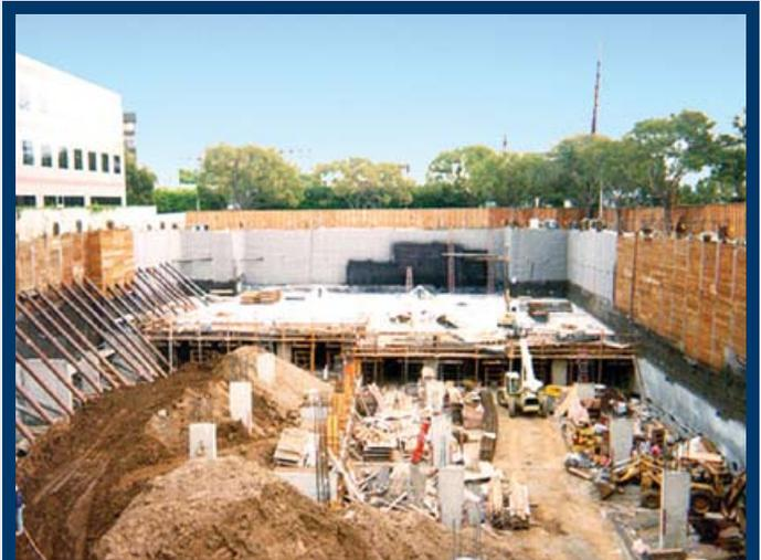
***The Universal Studios project needed a membrane that could withstand 750,000 gallons a day of groundwater. It needed to be tough enough that the shotcrete could be applied directly on its face.***
